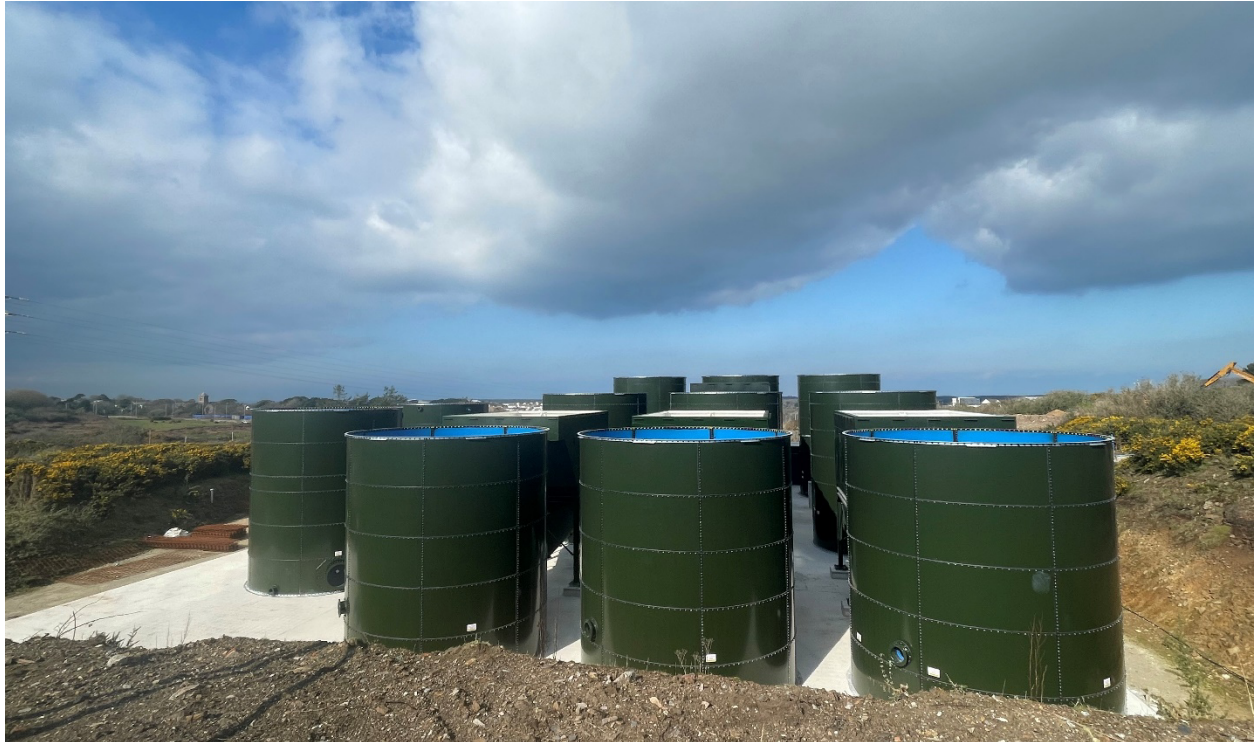
Photo 2 – The Water Treatment Plant as of March 2, 2023.
