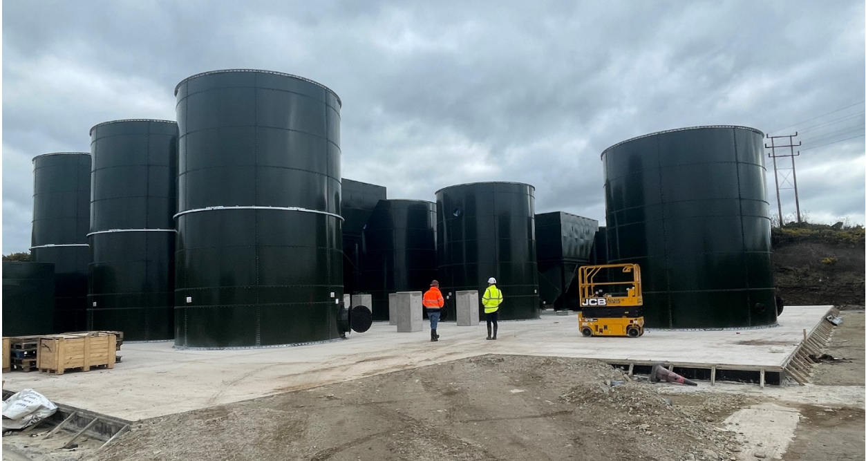
Photo 3 – Ground level view of the water treatment plant.
