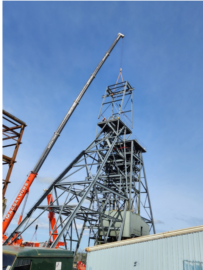
Removing the Gallows from NCK headframe
