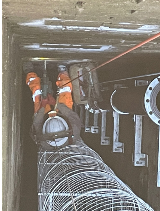
Installation of escape ladder and discharge pipes into Middle Engine Shaft
