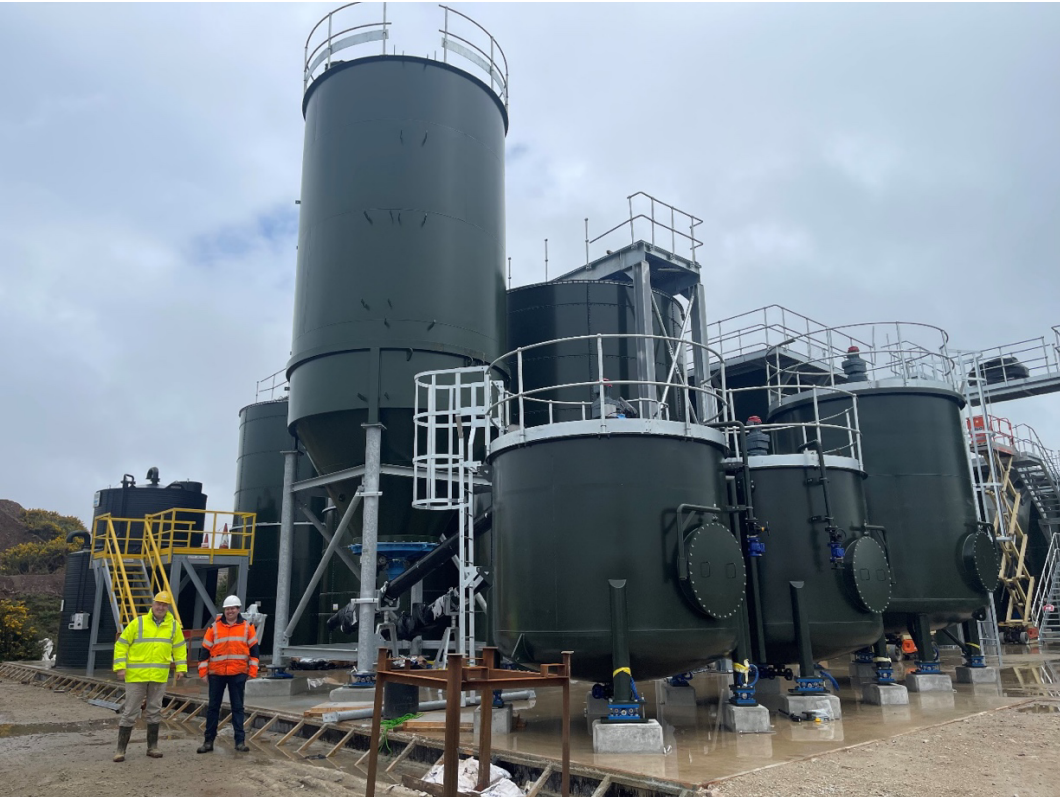
Side view of the water treatment plant looking southeast.
