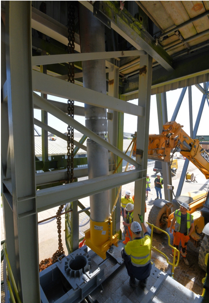
Photo 2. Positioning the submersible pump over the installation guide at NCK shaft.
