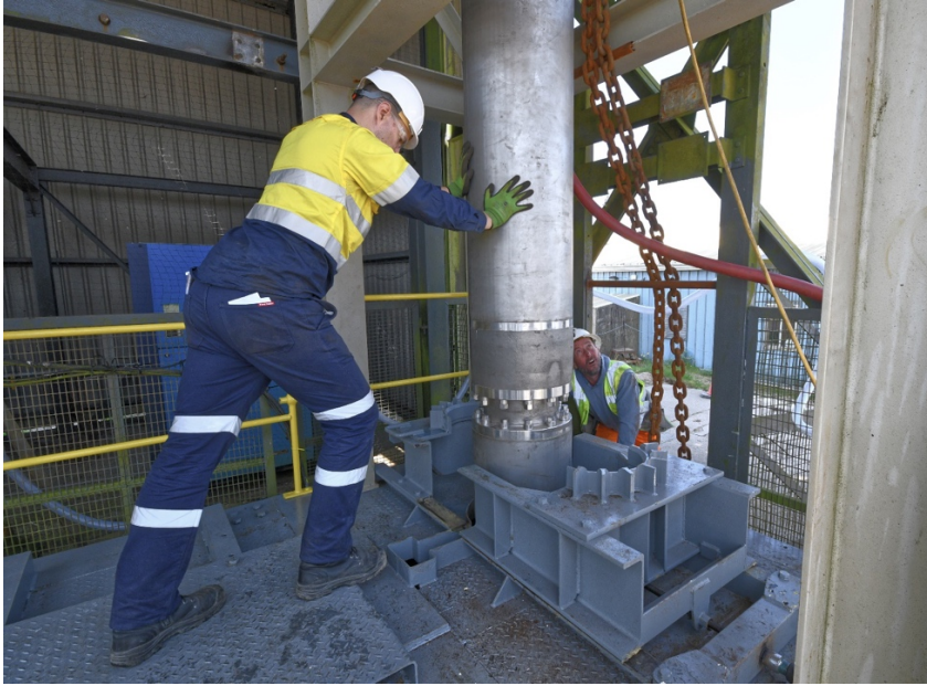
Photo 3. The submersible pump being lowered into NCK shaft.
