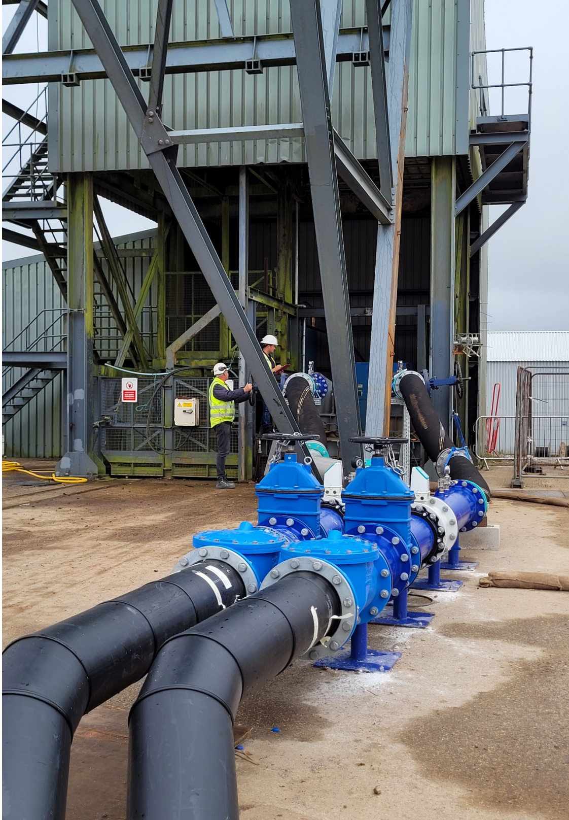
Photo 2 – Manifold completion at NCK shaft.
